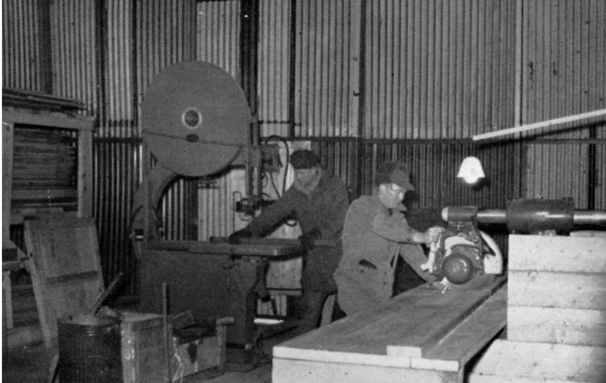
Carpenter shop (USAF photo)
